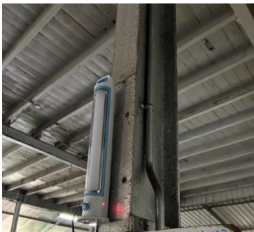
Installation of emergency lighting equipment
